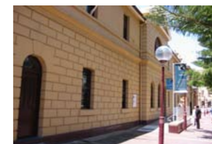
The Newcastle Police Station building was constructed in 1861 and is now a museum presenting the region's history of law and order. It is part of the complex managed by the Newcastle Historic Reserve Trust.
